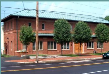
Appalachian Crossroads main building
